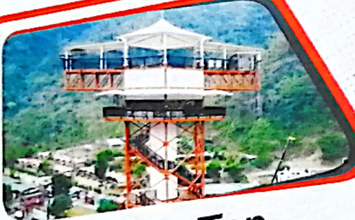
Tower Top Restaurant
